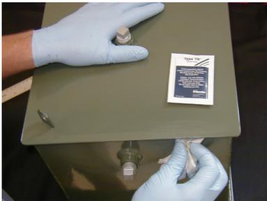
Clean area with cleaning wipe before applying PowerPatch<sup>®</sup> Putty
